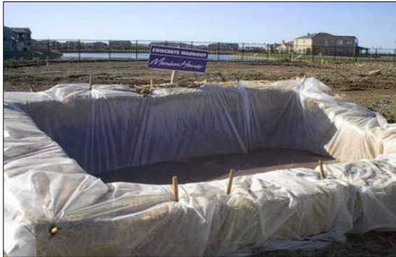
Plate 5-12 Concrete Washout Area
