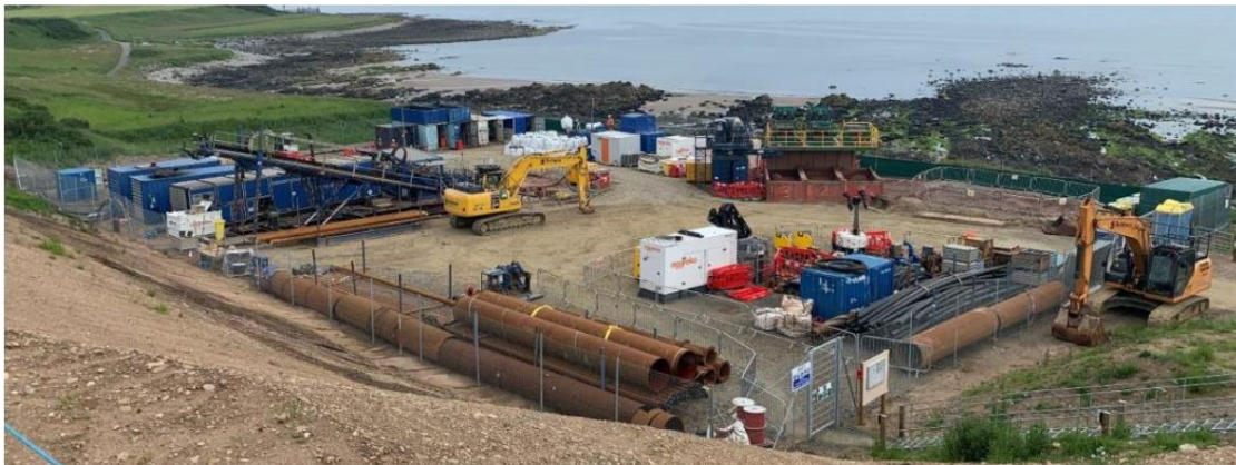
Plate 5-11 Example HDD compound
