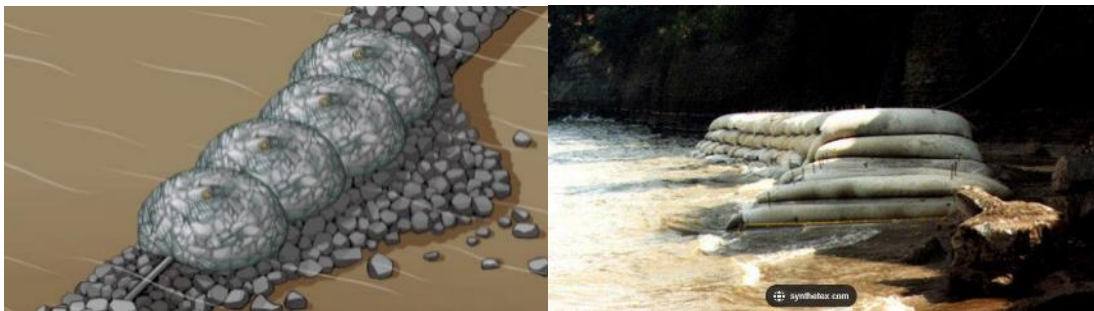
Plate 5-9 Rock bags (left) and grout bags (right) used as cable protection
